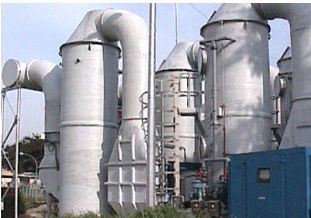
Chemical Scrubber for H2S Removal Singapore Sewage Treatment Plant
