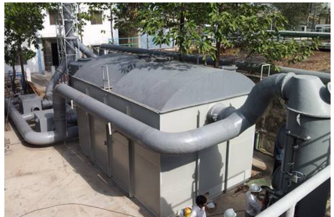
BioFilter for H2S Removal, AB Mauri, Vietnam
