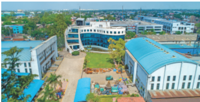
Unit 1, Indore with built up area spanning over 125,000 Sq. feet
