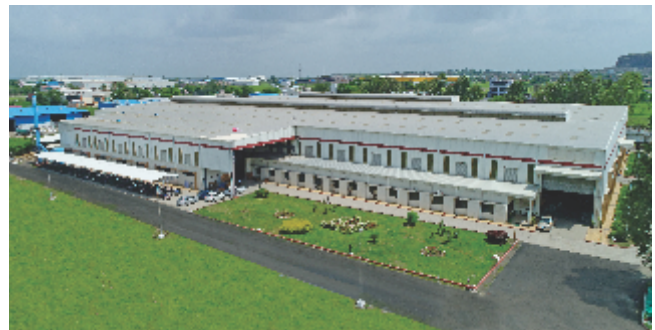
Unit 2, Indore with built up area spanning over 155,000 Sq. feet
